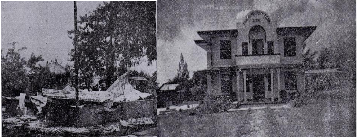
Figure 1. Old Municipal Building
